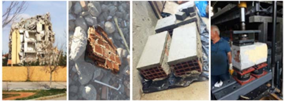
Figure A. Process of the research: Demolition, visual investigation, preparation for reuse, and testing
